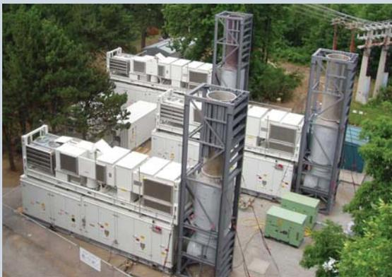
■ Three SGT-300 industrial gas turbine generator packages installed at a site in Canada to provide a reliable source of power. The units were supplied from stock and installed to allow operation within days of arrival.
