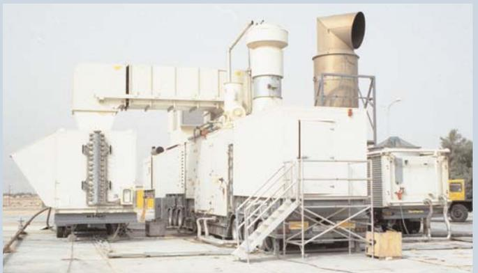
■ Four SGT-400 mobile packages operate in the Middle East, providing power to the local grid system. The units are capable of operation on either natural gas or diesel fuel and include the Siemens Dry Low Emission combustion technology. Each 13 MW mobile package is contained on four trailer units and includes a control room with switchgear, black start diesel and instrument air compressor.
